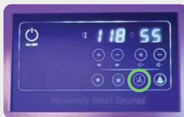
Heaters On / Off
