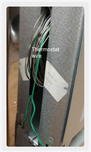
Run the thermostat wire up the wall and away from the heater at least 12 inches. The bulb should be mounted 12" - 24" from the ceiling of the sauna. Cover the thermostat wire with the wooden cover provided with the heater.
