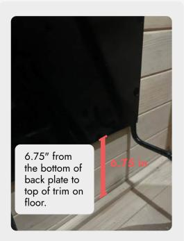
6.75 inches from the bottom of back plate to top of trim on floor.
